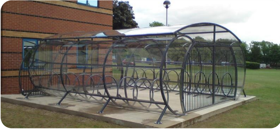
Above: Phase 2, Canopy 1
