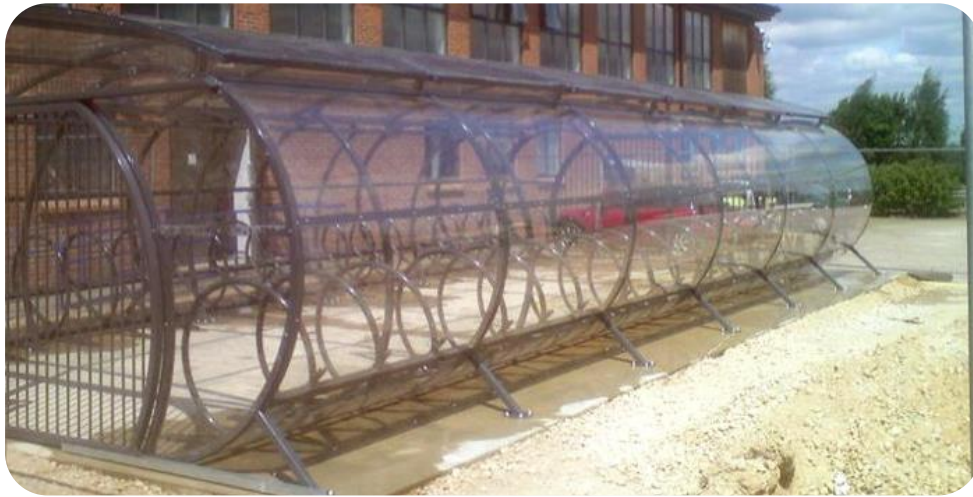
Above: Phase 2, Canopy 2
