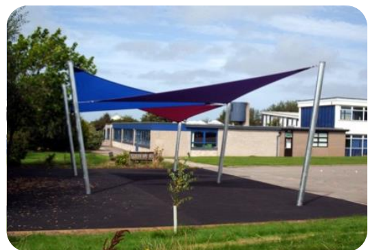
Above: The Installed Shade Sails
