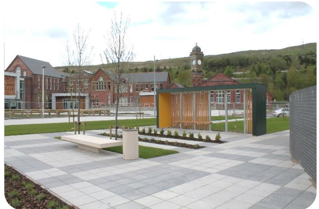
Above & Below: After Shelter Installation
